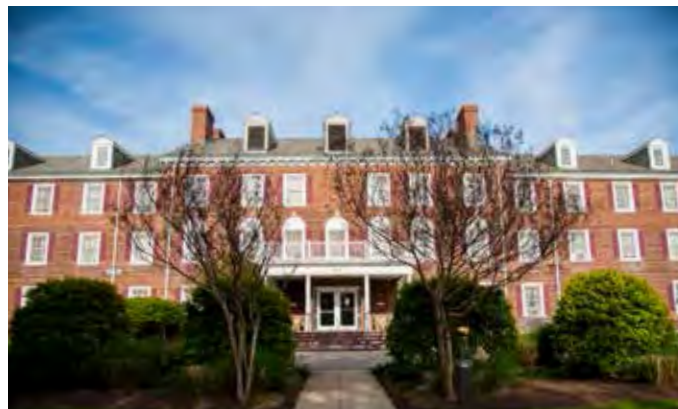
Original National Lutheran Home at 18 th & Douglas Streets, N.E., Washington, D.C.
